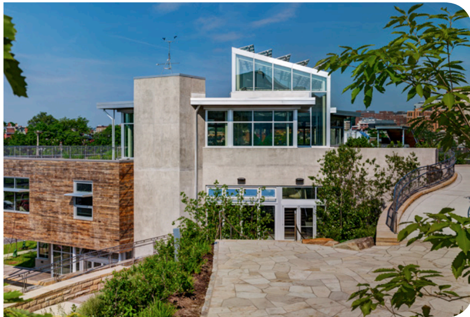
Sungate® 500 /Clear glass combined with Starphire® and Solarban® 60/Starphire® glasses were specified for the Center for Sustainable Landscapes at Phipps Conservatory and Botanical Gardens, with the goal of satisfying the requirements of the Living Building Challenge. The building is also designed to meet LEED® Platinum certification for sustainable design and SITES certification for landscapes.
